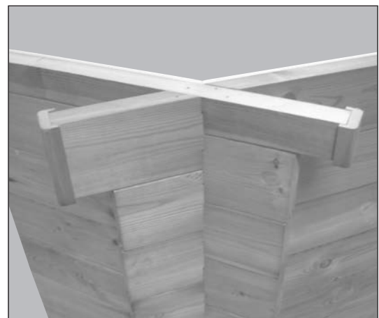
Figure 4. Top of Wall.
