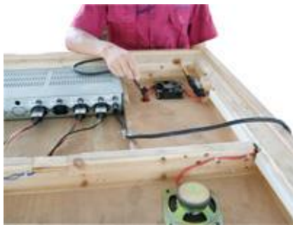
FIG-17 Put down the wires into the sauna cabin
