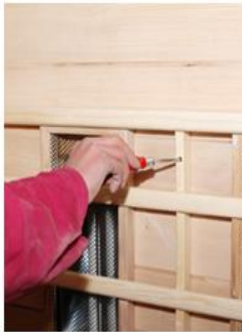
FIG-12 Assembling front board
