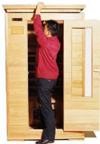
FIG-14 Setting the top board
