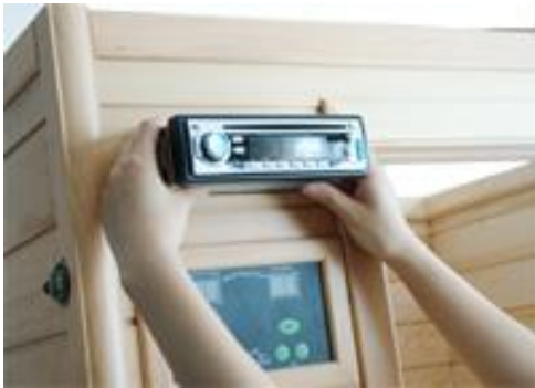
FIG- 13.1 Fixing stereo w/ CD
