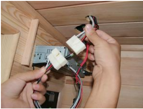
FIG-18 Link the CD connectors
